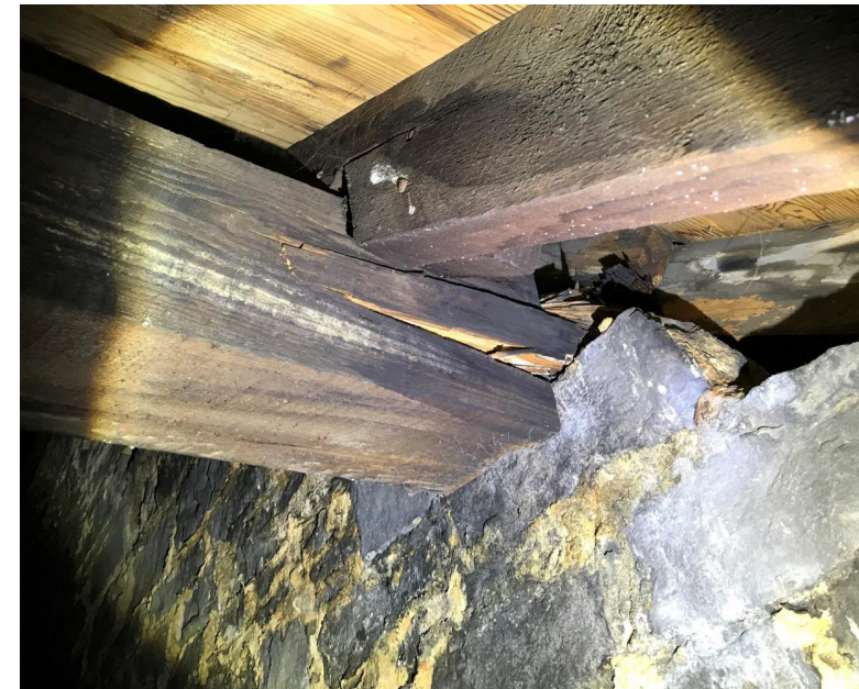
Significant split at the end of main support beam, 3"-4" drop causing weight shift to roof rafters
