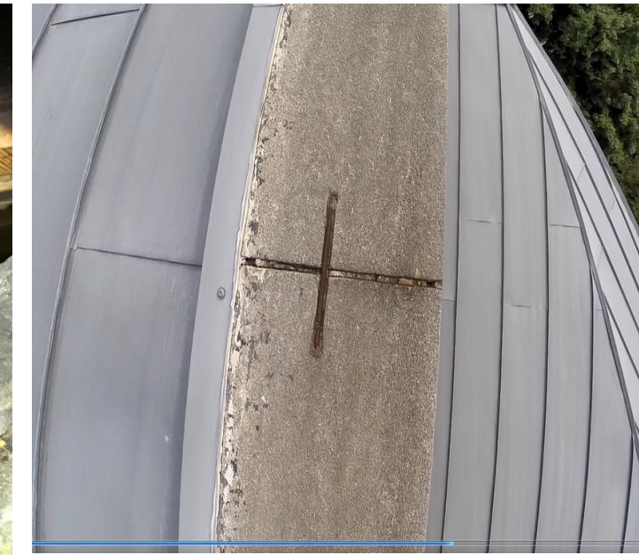
Missing and cracked mortar on rooftop
