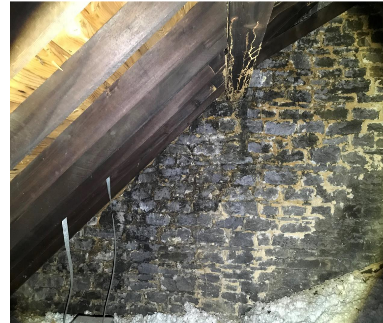
Significant split at the end of main support beam, 3"-4" drop causing weight shift to roof rafters
